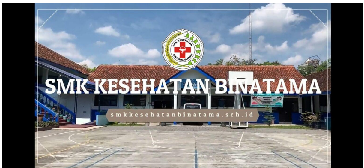
Gambar 1. SMK Binatama Jalan Monjali, Sleman, DIY
